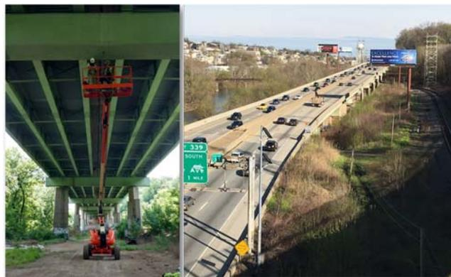
Figure 3. Operational Monitoring Application to a RC Deck-on-Steel Girders Viaduct
