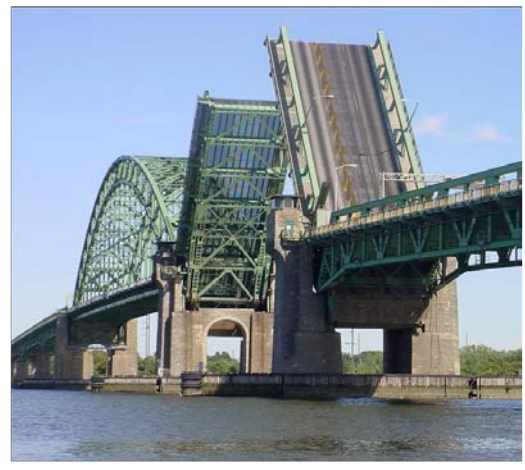
Figure 1: The Tacony-Palmyra Bridge
